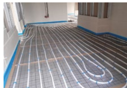
... and a view of the inside during installation of the floor heating.
